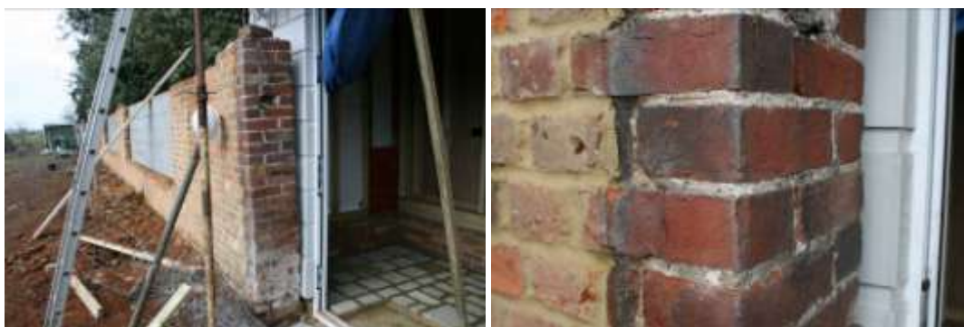
The brick remnant of the garden wall and detail of the penny struck pointing.
