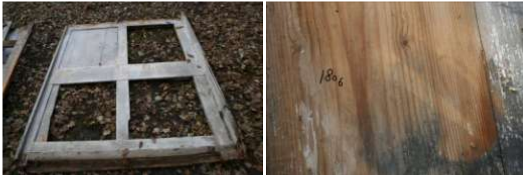
Original phase panelling with heavy section timbers dated 1806. (Overlined).
