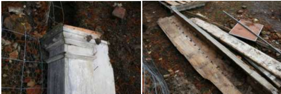
The capital of the regency style pilaster and the interior construction showing the fillets
