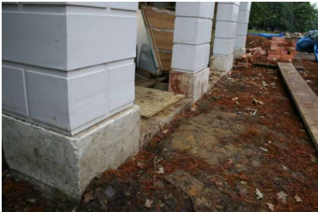
Original ashlar block pediments and stone door cills set on a brick plinth. Looking W.
