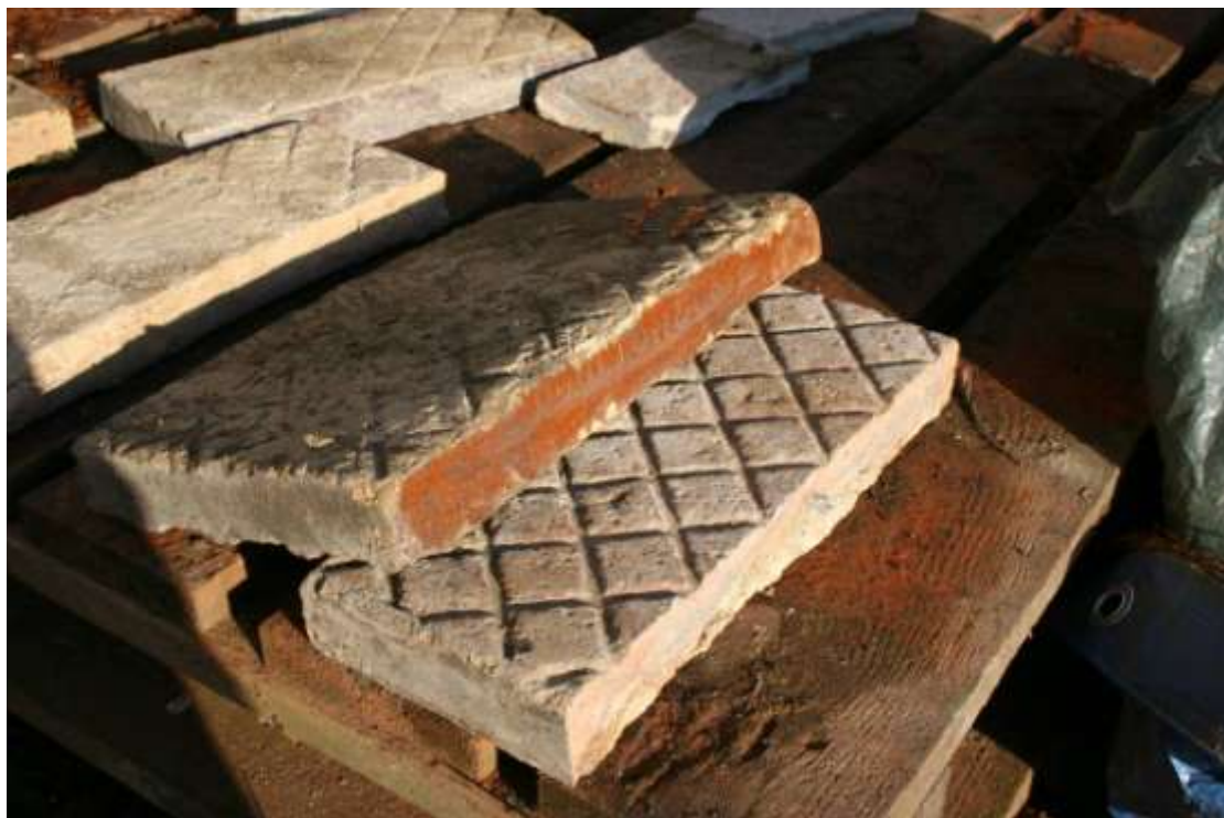
Doulton & Co ceramic floor tiles used in the rear of the building.
