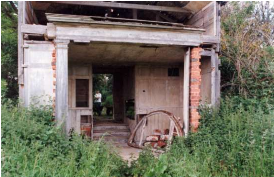
November 1997 showing the regency pilaster in-situ and the early basculating window.
