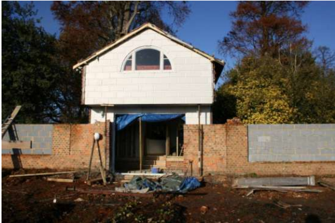
The southern elevation has a replica window and applied rustication.
