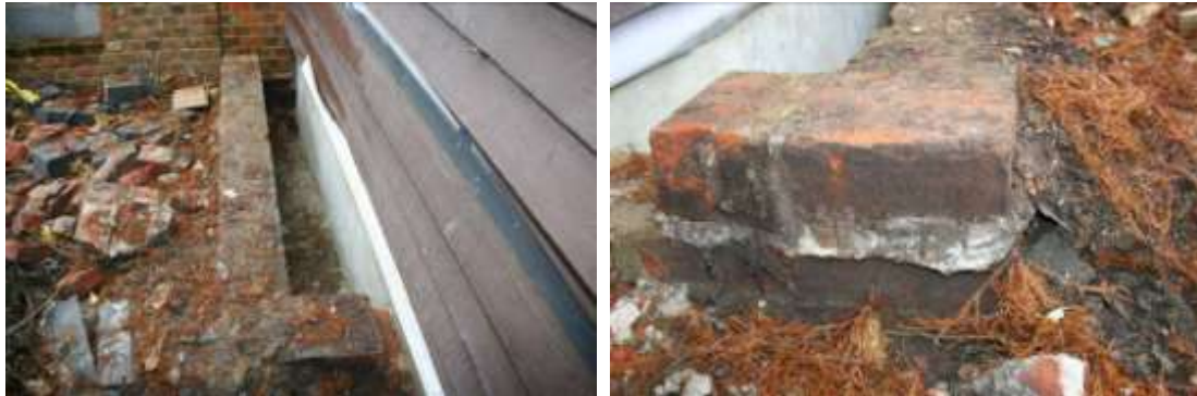
Brick plinths either side of the Summerhouse. Detail of the soldier course and white mortar.
