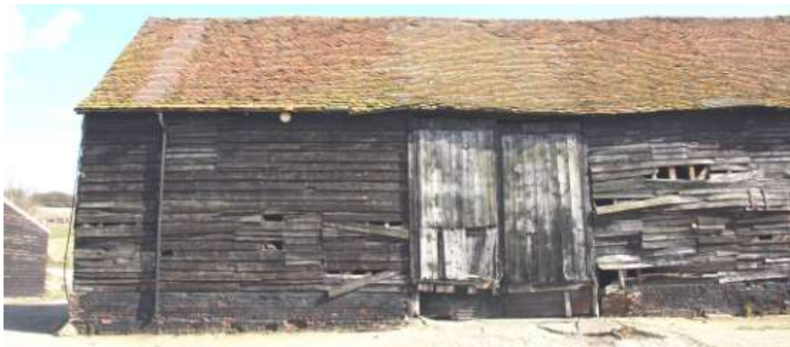
The position of redundant windows is denoted by short sections of modern weatherboards.
