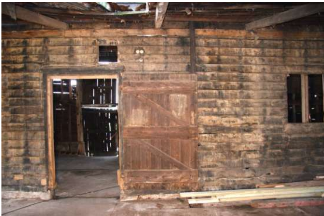
The eastern elevation of the barn inside the Chicken House. C20th door and unframed window.
