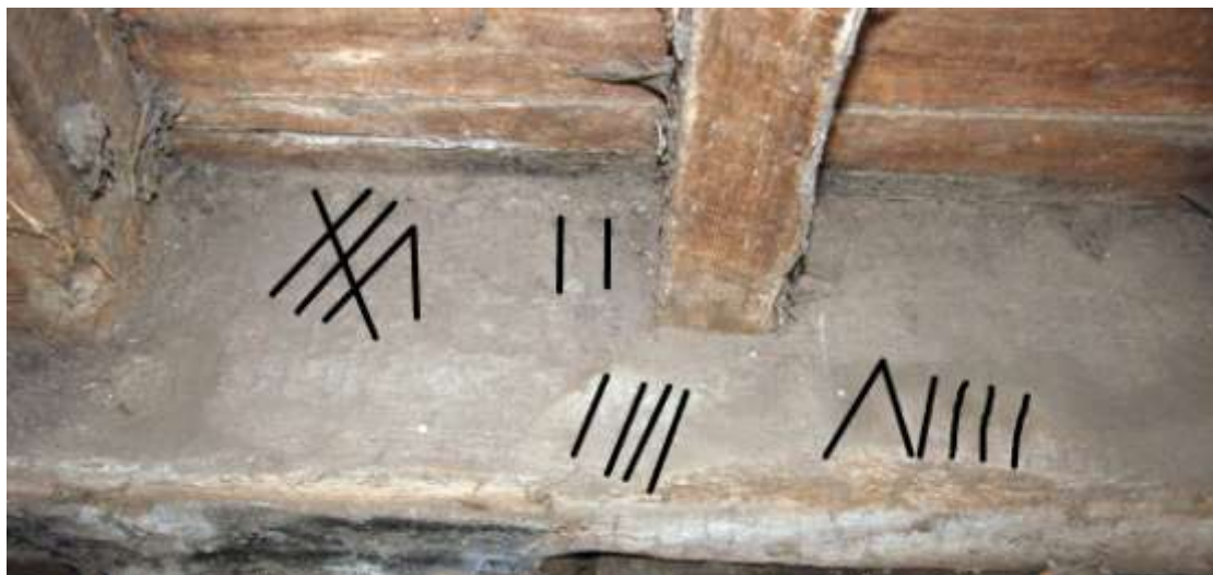
Carpenter's marks on the softwood sole plate in Bay 6. Enhanced in Photoshop CS2.
