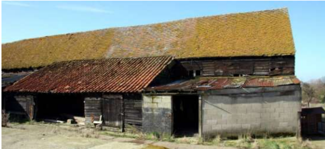
The Flat-roofed Outshot from the east showing the tin roof and breeze block wall.
