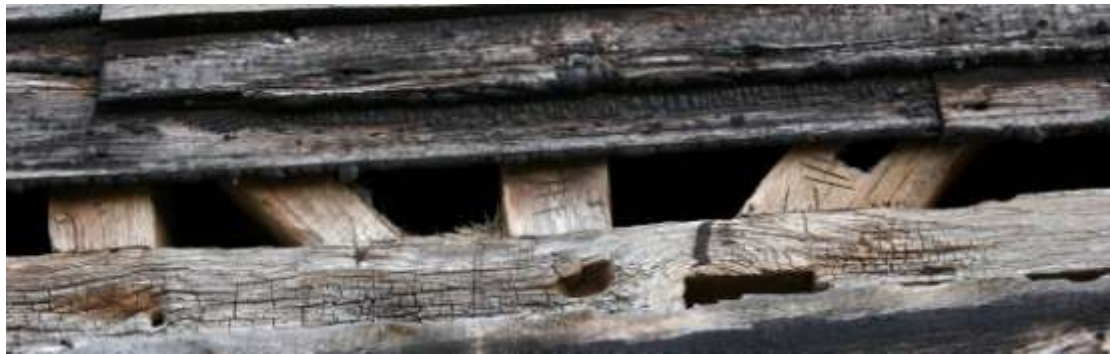
Carpenter's marks on the western elevation.
