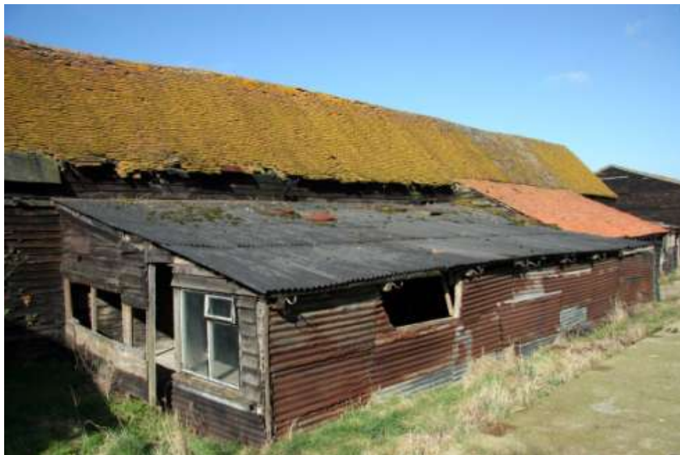
The Chicken House on the eastern elevation of the barn.
