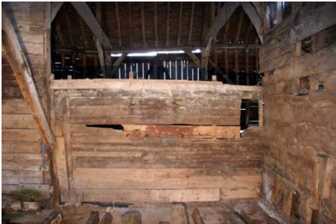
C20th vernacular partition between the barn and the Central Outshot constructed by Mr Chapman senior.
