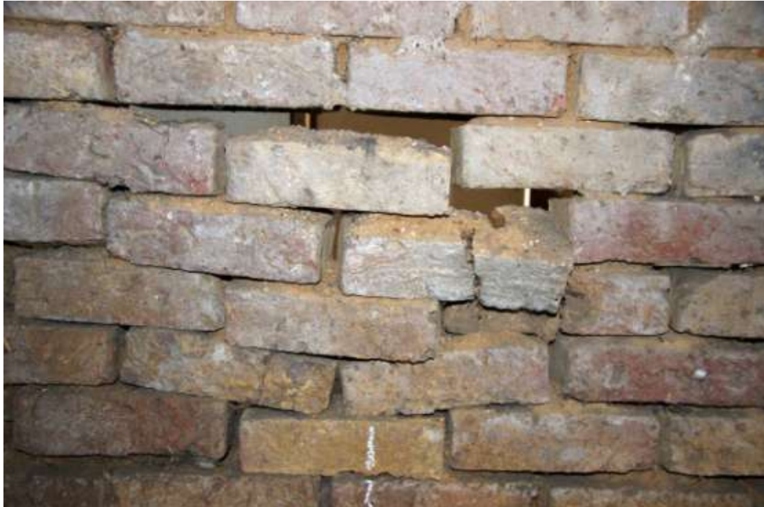
The failing pointing in the northern wall of the Cleaning Room.
