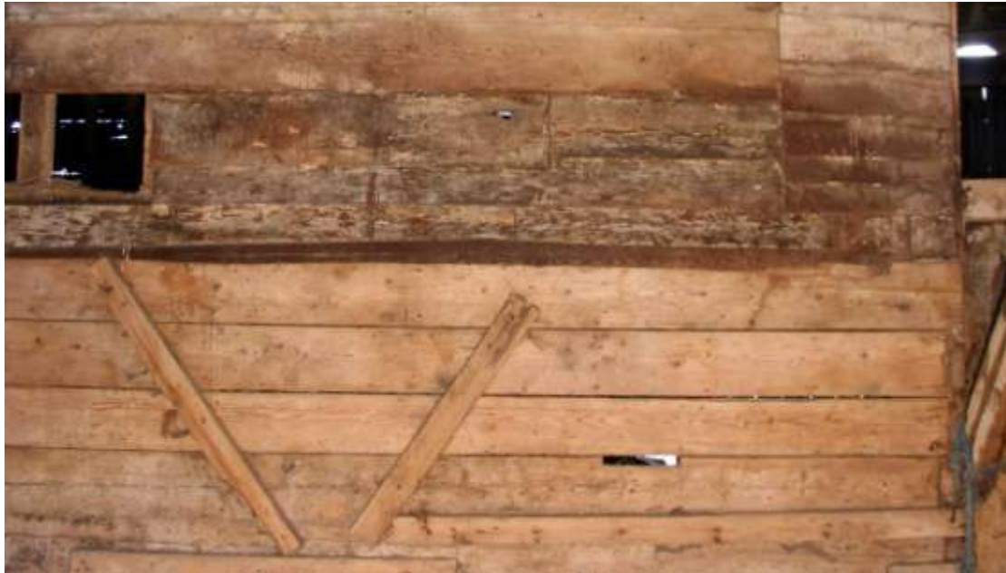
Manger support rails are nailed to the floorboards applied by Mr Chapman senior.
