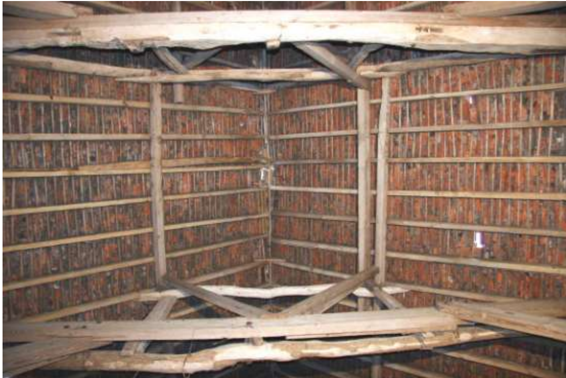
Bay 9 looking south showing trusses 8 and 9. Note the double purlin to the western side and the old poles doubled up with C20th timber.
