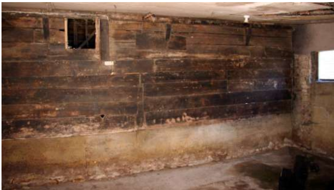
The weather boarding is made of reused floorboards put in in the C20th.
