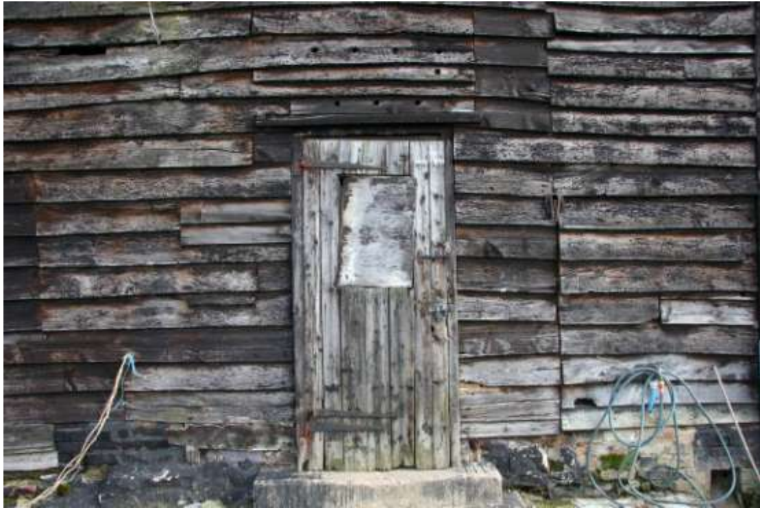
The C20th door into the Cleaning Room.
