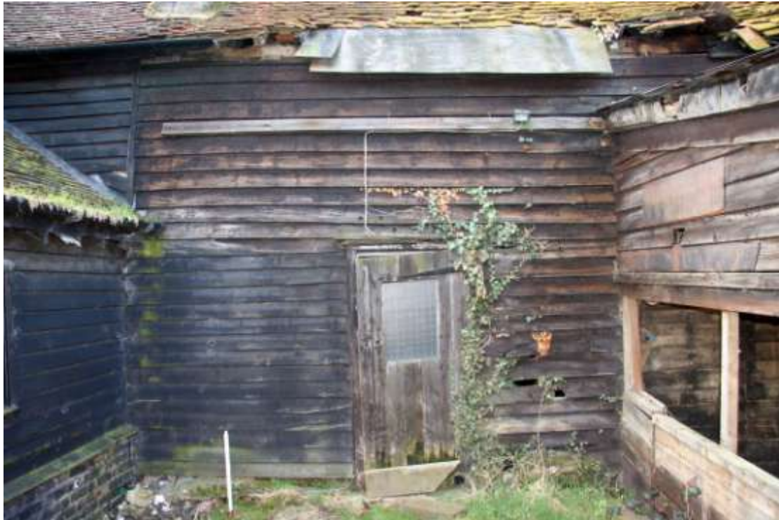
The back door to the Cleaning Room. Weatherboarding and door are C20th.
